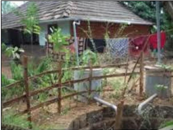
Example of a typical Rooftop RWH Open Well Recharge system, setup under the Mazhapolima program, at a home in Thrissur district.
